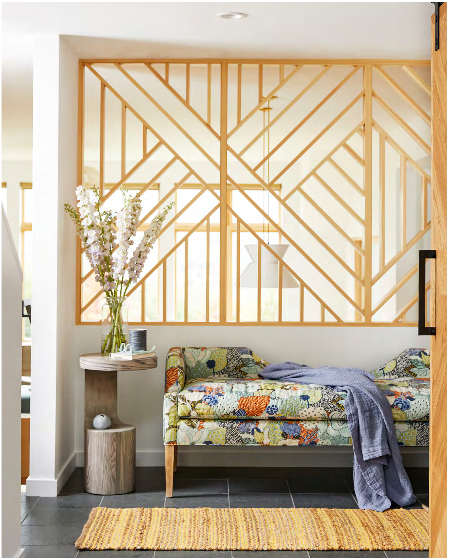
A decorative screen takes the place of a closet in the entry to allow for natural light and mountain views. "We thought about installing a window, but I played around and came up with this three-panel design that the builder executed in clear pine," says designer Teri Maher. PHOTOGRAPH BY LIZ DALY/STYLING BY MELAÑIO GOMEZ
