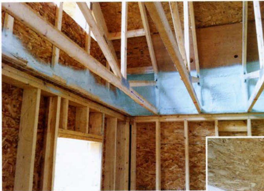
Figure 6. The truss heels and other framing joints were first air-sealed with closed-cell foam in preparation for blown-in cellulose (left). Note the site-built baffles behind the foam — pieces of plywood over strips of wood along the top chords — which allowed for 30 inches of insulation without blocking the soffit vents. To support all that cellulose, the author installed OSB rather than drywall on the bottom chords of the trusses (below). Sealed with tape and mud, the OSB provides an airtight seal between conditioned space and the attic and solid backing for the tongue-and-groove wood ceiling that followed.
