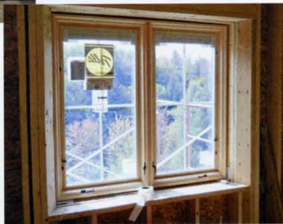
Figure 5. After the exterior stud bays were sprayed with 3½ inches of closed-cell foam, workers let in blocking for a future addition, then covered the foamed stud bays with housewrap (above left). The windows are fastened directly to the bucks, then flashed to the housewrap with flashing tape (left). The window openings were framed with a 30-degree flare to allow in more light (above).
