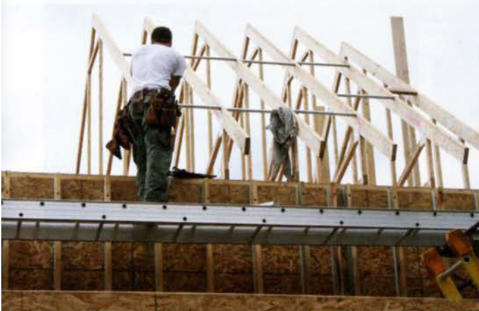
Figure 4. The roof was framed with raised-heel trusses, which allow for 24 inches of blown cellulose under the top chords at the plates (above). The trusses also have raised bottom chords down the center, creating a comfortable passageway and work platform for mechanical contractors. Dropped gable trusses support the 2½-foot-deep gable overhangs, shown here being blocked (right).
