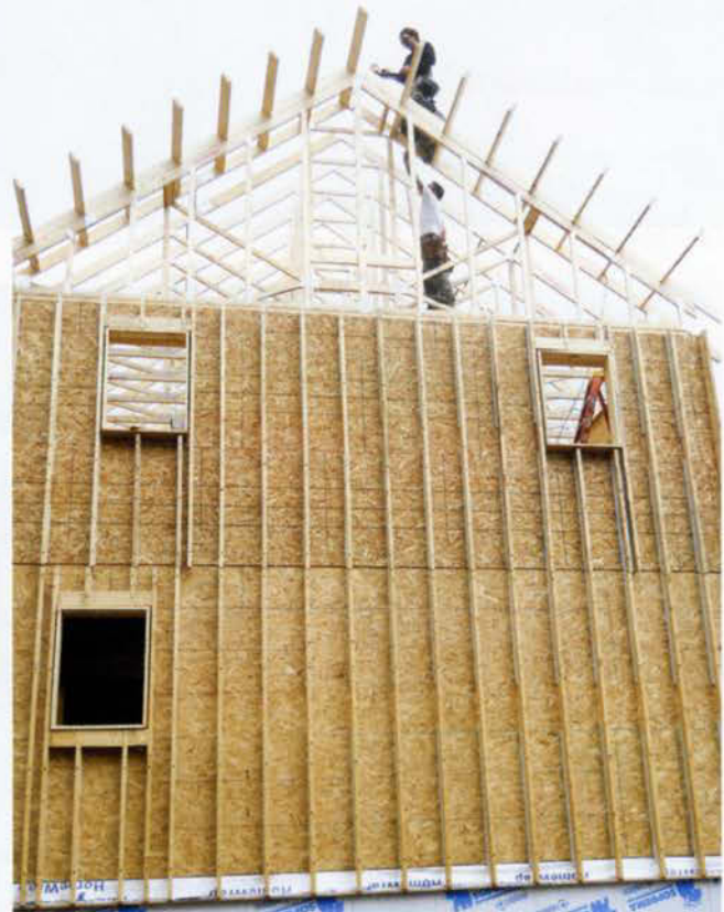
Figure 4. The roof was framed with raised-heel trusses, which allow for 24 inches of blown cellulose under the top chords at the plates (above). The trusses also have raised bottom chords down the center, creating a comfortable passageway and work platform for mechanical contractors. Dropped gable trusses support the 2½-foot-deep gable overhangs, shown here being blocked (right).
