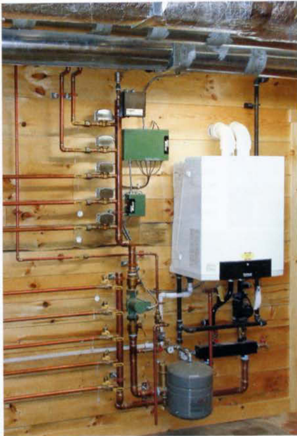
Figure 7. The home's heat is supplied by a Buderus wall-mounted propane boiler (above). The condensing unit has variable output between 22,500 and 75,000 Btu, depending on how many of the five zones are calling for heat. The 80-gallon Superstor Solar storage tank (above right) receives hot water from two roof-mounted solar thermal collectors (right); backup is provided by an electric heating element. To the left of the storage tank is a Venmar EKO 1.5 heat-recovery ventilator.
