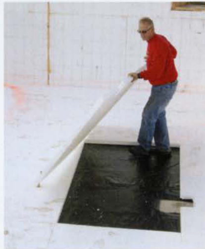
Figure 1. Fabric footing forms remain in place after the concrete is poured, creating a capillary break between the ground and the footing (top). R-26 ICF forms were used to build the foundation walls (above), which were wrapped with an additional 2-inch layer of EPS, then waterproofed with a foundation-grade peel-and-stick membrane (far left). The basement slab is insulated with two layers of 2-inch EPS foam, with a vapor barrier sandwiched in between (left).
