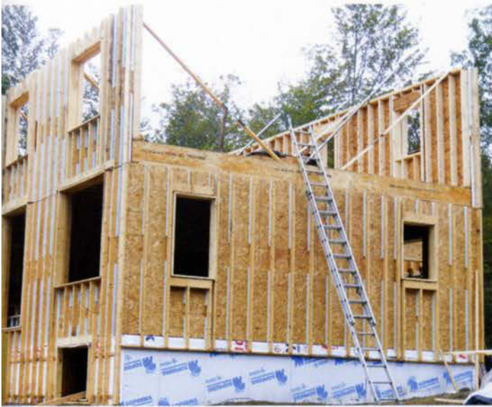
Figure 3. The exterior walls were framed so that, when lifted into place, the OSB sheathing and the outer 2x4 studs cover the rim joists (left), providing continuous bays for spray foam from the foundation to the truss top chords (below).
