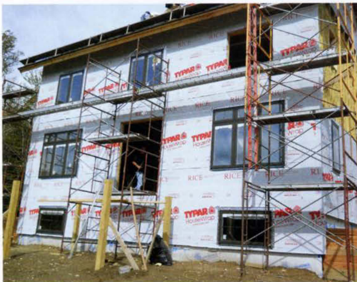
Figure 5. After the exterior stud bays were sprayed with 3½ inches of closed-cell foam, workers let in blocking for a future addition, then covered the foamed stud bays with housewrap (above left). The windows are fastened directly to the bucks, then flashed to the housewrap with flashing tape (left). The window openings were framed with a 30-degree flare to allow in more light (above).
