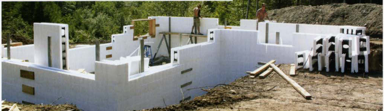
Figure 1. Fabric footing forms remain in place after the concrete is poured, creating a capillary break between the ground and the footing (top). R-26 ICF forms were used to build the foundation walls (above), which were wrapped with an additional 2-inch layer of EPS, then waterproofed with a foundation-grade peel-and-stick membrane (far left). The basement slab is insulated with two layers of 2-inch EPS foam, with a vapor barrier sandwiched in between (left).
