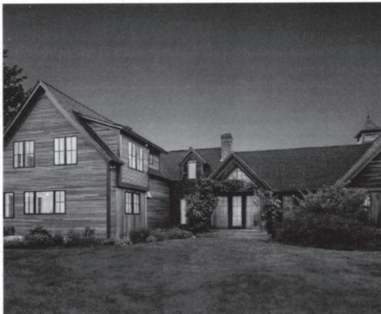
New School Builders received an award for Best Residential Renovation in the $251,000 to $400,000 category.
